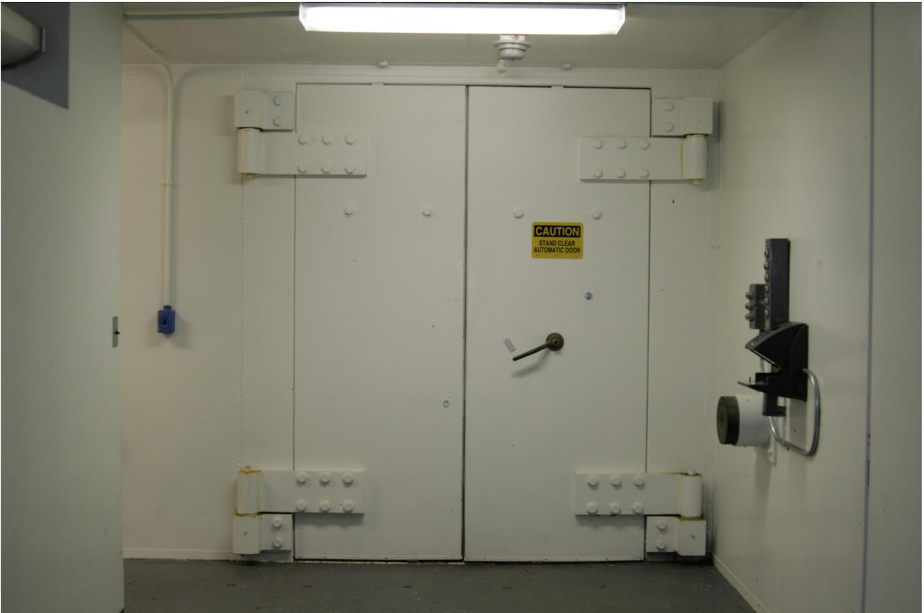
These 3000 lb solid steel blast doors are capable of withstanding the enormous overpressure of a nuclear detonation within 2 miles. This over-engineering means that the doors exceed even the heaviest bank vault standards and are essentially impenetrable.
